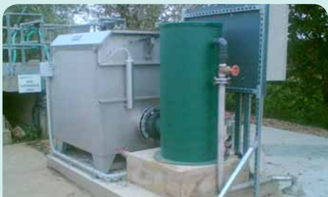
Site: Great Horwood | Anglian Water | 34 l/s site
