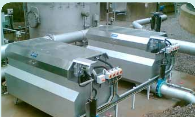
Site: Shepton Mallett | Wessex Water | 136 l/s site
