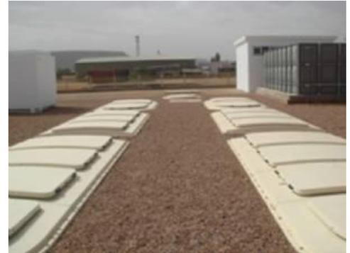
WPL provided a new bespoke HiPAF (High Performance Aerated Filter) plant to sit alongside the previous system they provided to the site located in a remote part of south western Libya. When providing the new sewage treatment solution WPL modernised the prior system to bring it up to date with current Libyan and World Health Organisation (WHO) irrigation regulations and to treat the wastewater to the highest international standards.
