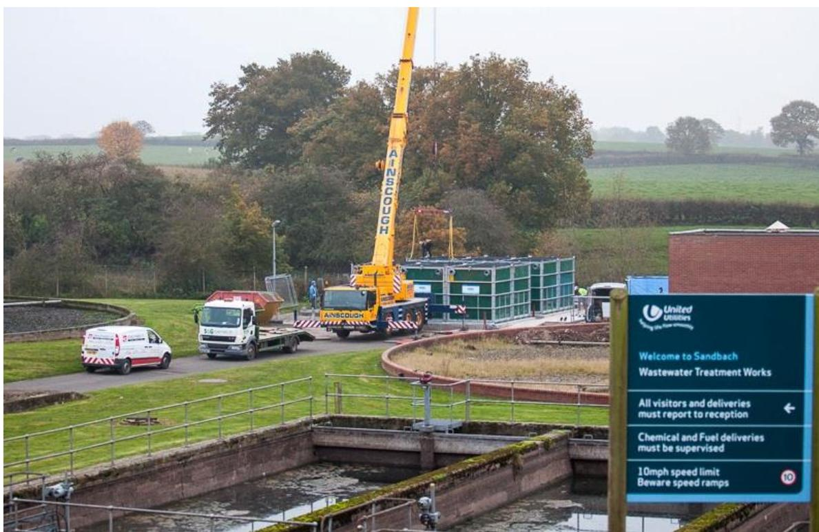
WPL Hybrid-SAF units can operate as individual treatment plants or the modular design means they can be connected in series to form larger plants. The plants are built offsite in a specially controlled environment, which minimizes the time required for onsite installation.
