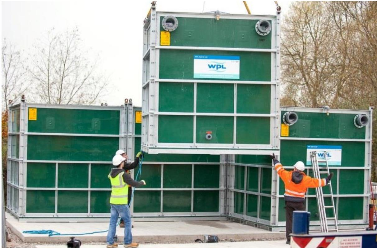
The modular nature of the WPL Hybrid-SAF means units can be installed even where sites face height and width constraints. In certain circumstances, WPL can increase the height or width of individual units at the design stage to accommodate site constraints.
