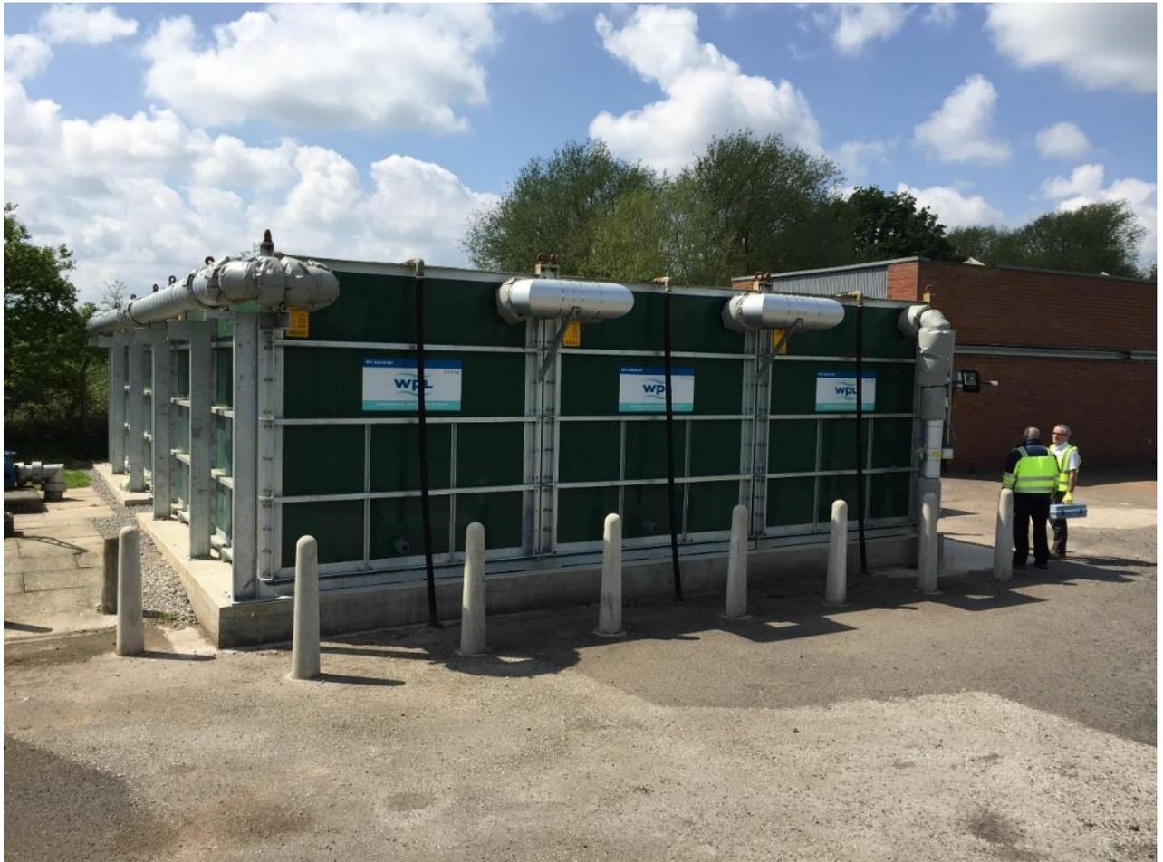
UK manufacturer WPL has installed enhanced models of its Hybrid-SAF™ (submerged aerated filter) modular wastewater treatment plants at two United Utilities (UU) sites - Sandbach in Cheshire and Lawton Gate in Staffordshire.
